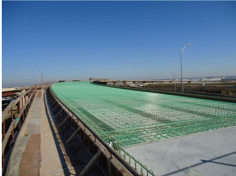
Deck work on the westbound SH 114 to southbound International Parkway Bridge.
