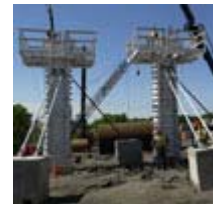
Bridge construction north of the DFW Airport
