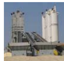
Concrete batch plant north of SH 114/121
