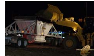
Night grading work at Main Street
