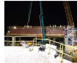
Bridge work north of DFW Airport
